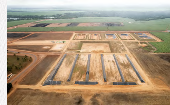
Construction of uisa Geo Biogas
