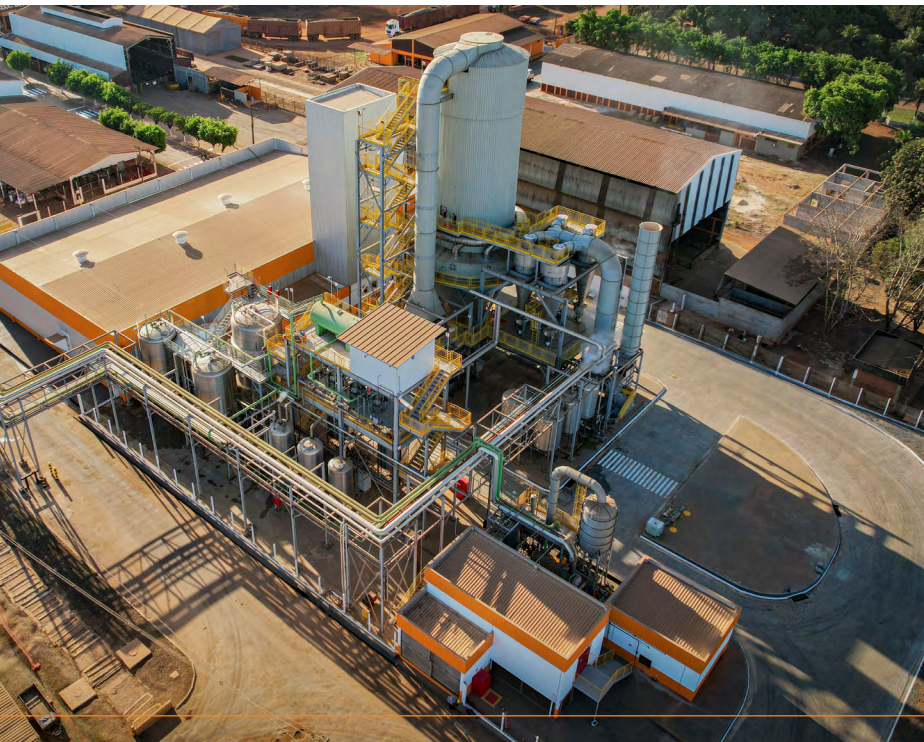
UISA BIONUTRITION, CONSTRUCTION COMPLETED
