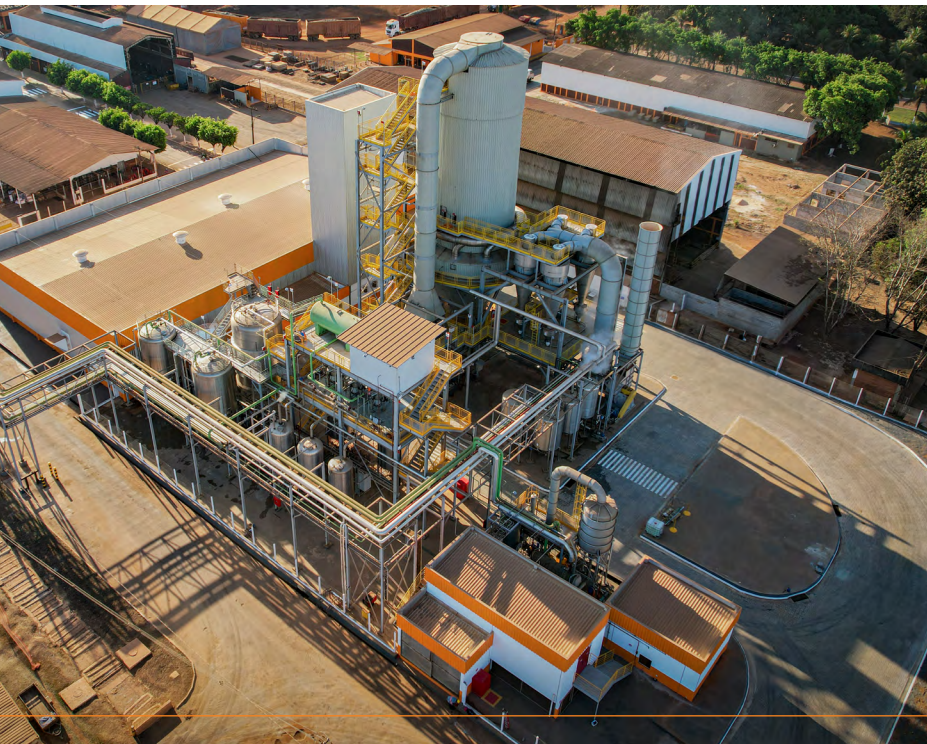
UISA BIONUTRITION, CONSTRUCTION COMPLETED
